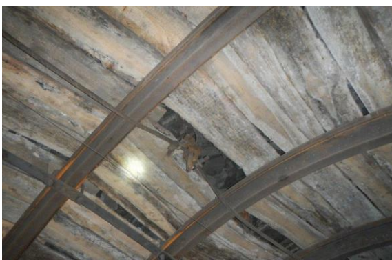
Figure 15. Fragment of the installation of rope crown runners at the experimental site of the 594 prefabricated drift, “Yuvileina” mine
