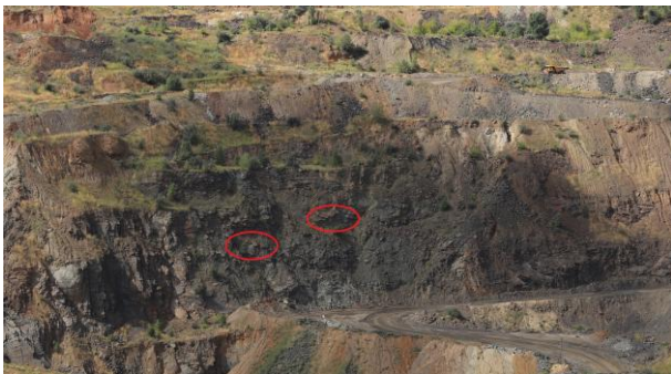
Figure 3. Location of two points on the steep slope of the eastern wall of quarry No. 4
