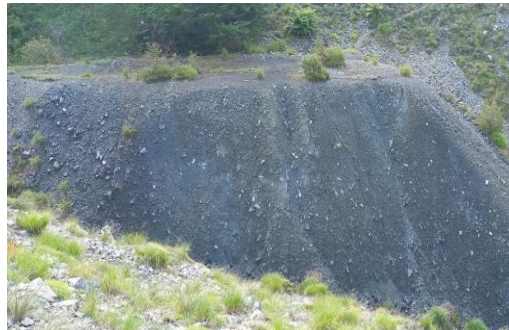
Figure 3. Remnants of asbestos-containing tailings and landfill sites in the Bajgora region are associated with historical mining activities since the 1940s
