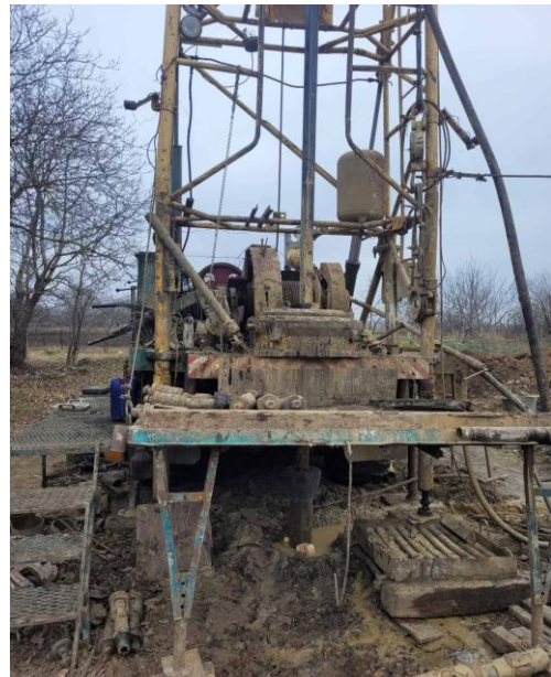
Figure 8. Well flushing through a filter column at the Veselinov area of Veselinivskiy district, Mykolaiv region
