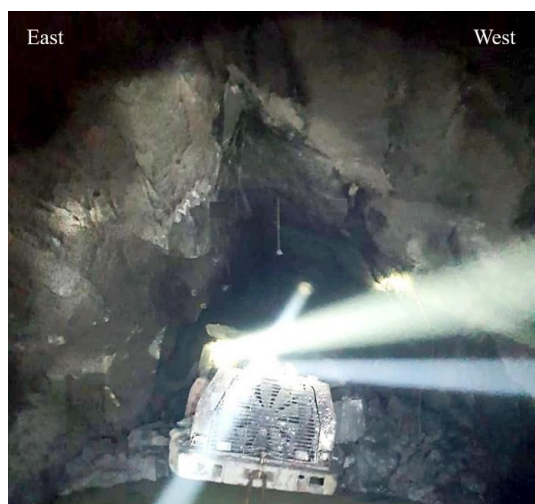
Figure 16. Wedge-shaped rockfall in a ventilation drift at 705 m horizon at the Shatyrkul mine on April 7, 2020
