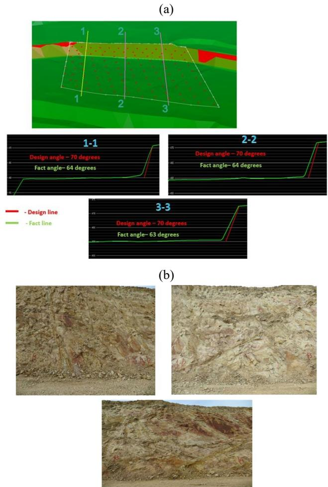
Figure 6. Effect of blasting the contour charges on the bench slope: (a) comparison of design and actual slope angles based on modeling results; (b) actual slope state after the blast at block 460-037
