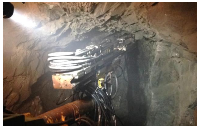
Figure 3. Drilling of injection wells
