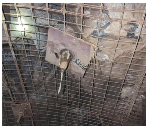
Figure 13. General view of the roof bolt after complete filling
