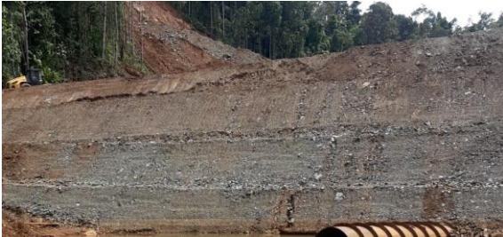
Figure 14. Embankment slope of STA 20 + 250
