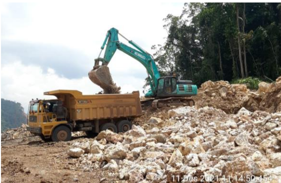
Figure 15. Embankment material for STA 20 + 250
